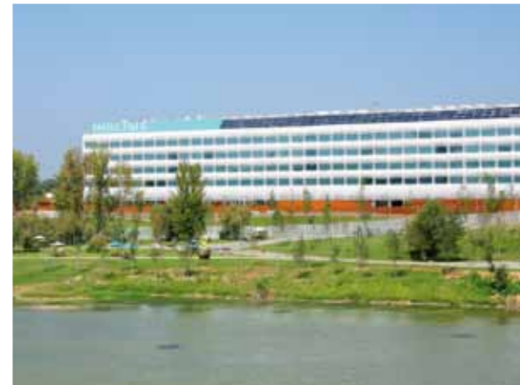
FACHADA HOTEL / HOTEL EXTERIOR
